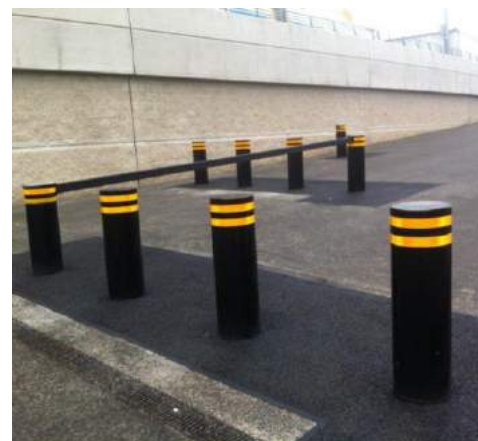
An example of a modified, fibre strap barrier for an undisclosed project
