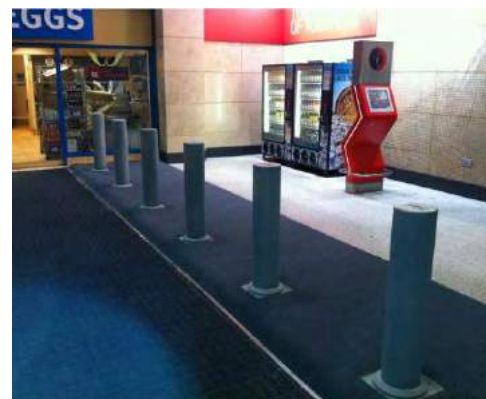
Surface Mounted Bollards Installed Inside a Shopping Centre
